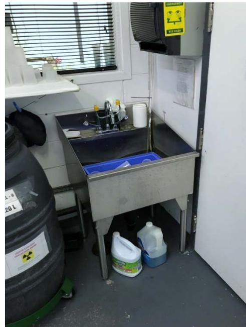
**Photo 2:** Eye wash station in the tritium laboratory area cleared of obstructions
