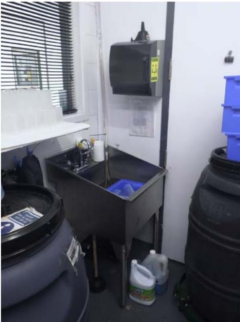
**Photo 1:** Obstructed eye wash station in the tritium laboratory area
