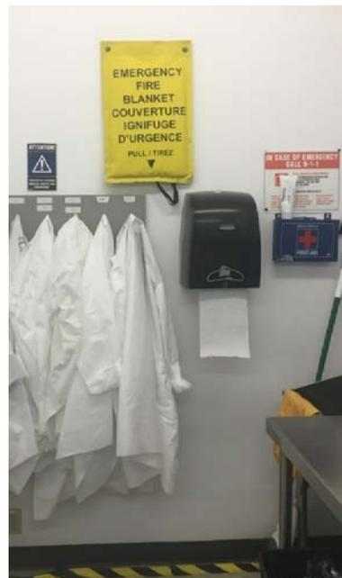
**Photo 3:** Obstructed fire blanket in the Coating room
