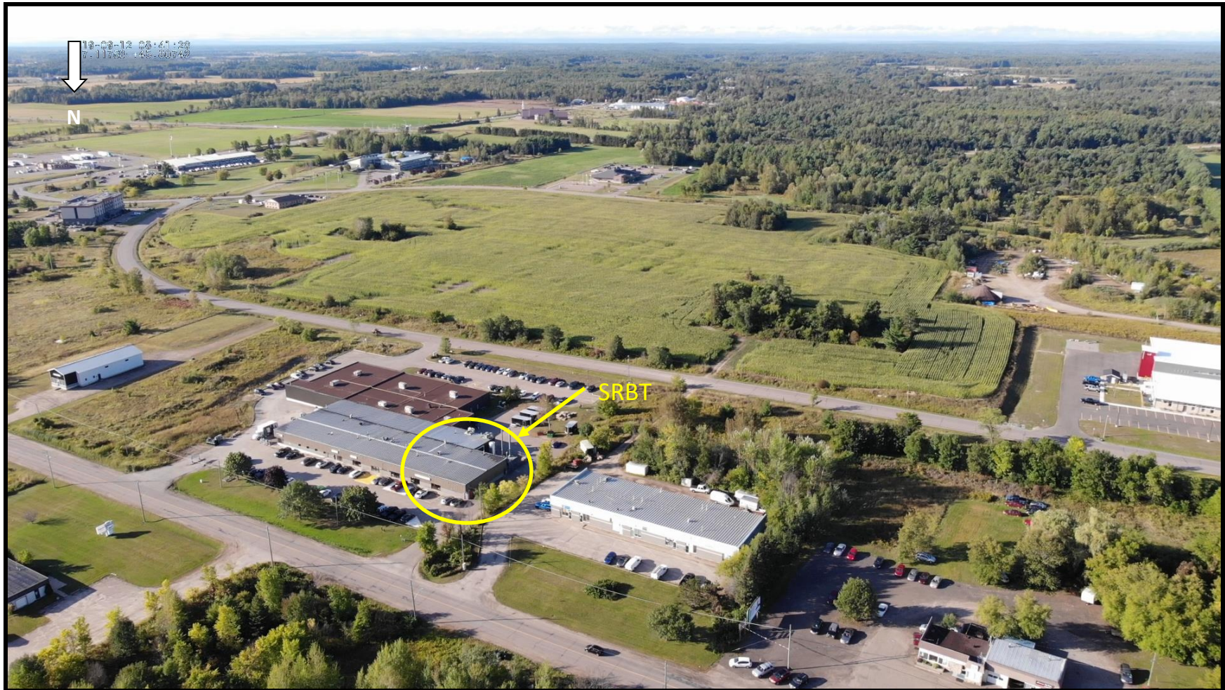
Figure 1.3: Aerial photograph of the SRBT facility
